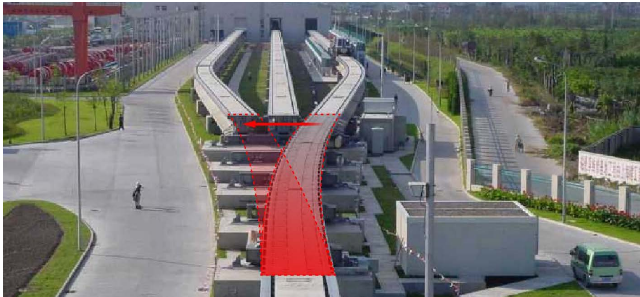
Figure 57. Transrapid guideway switch in Shanghai
