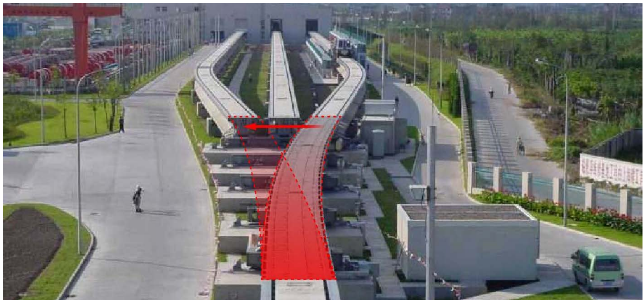
Figure 59. Transrapid guideway switch in Shanghai.
